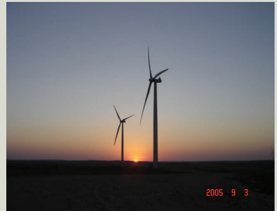
Ainsworth Wind Energy Facility
